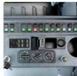
Centralized Instrument Switch Panel
